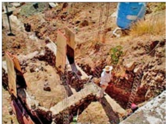
From above, as foundations go down
