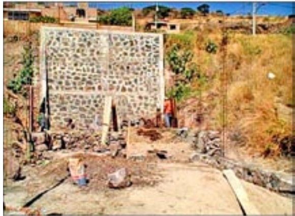
Retaining wall at the back of the property
