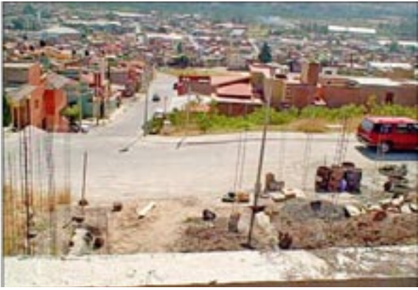
Prayer view from the top of the retaining wall
